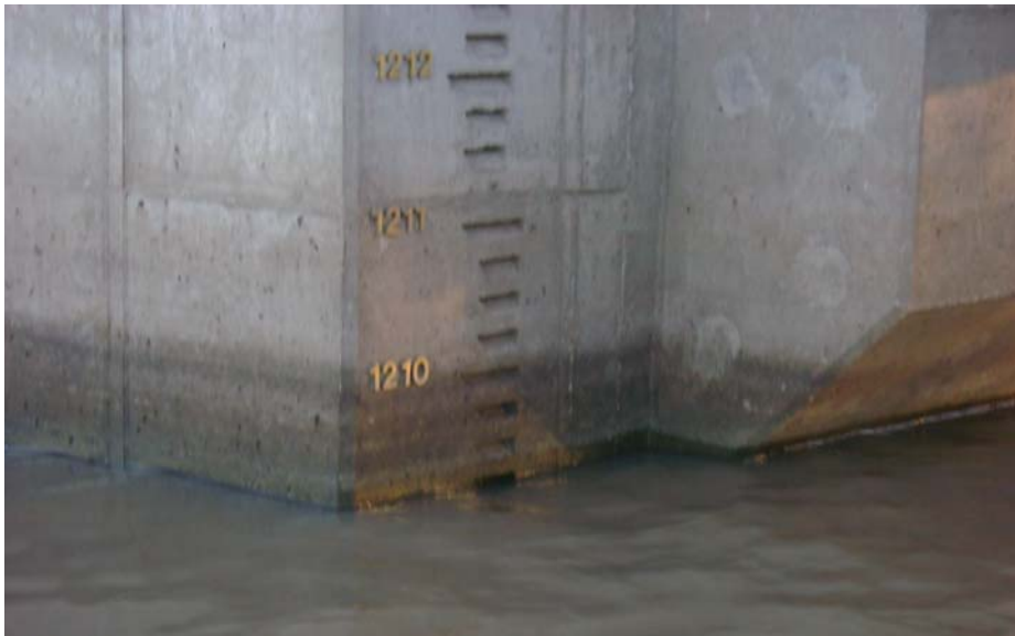
Figure 3a. Water surface elevation gauge on intake tower, Wellington Lake, November 15, 2007.
