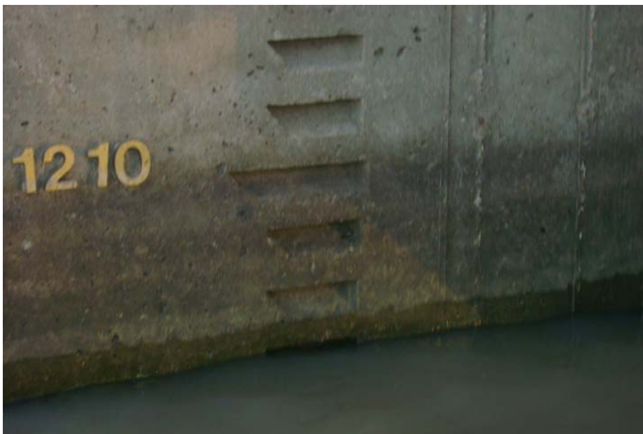
Figure 3b. Closeup: Water surface elevation gauge on intake tower, Wellington Lake, November 15, 2007. Water elevation is 1209.25 feet.
