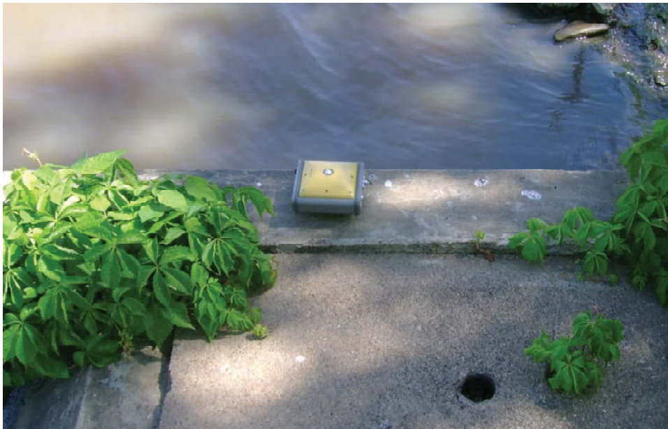
Figure 3b. Close-up view of lake elevation benchmark site.
