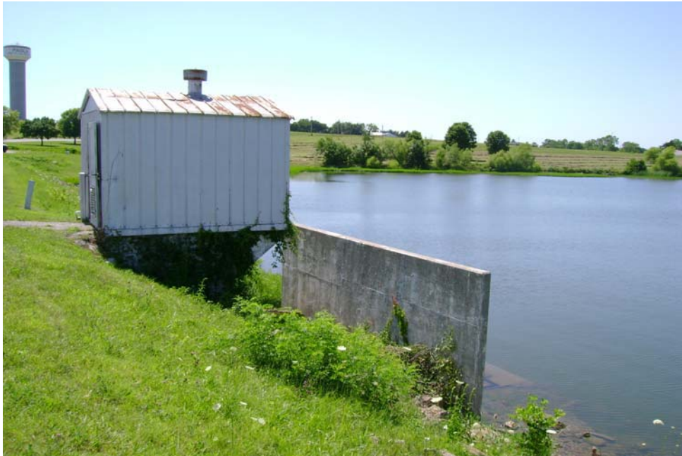
Figure 3a. View west along dam.
