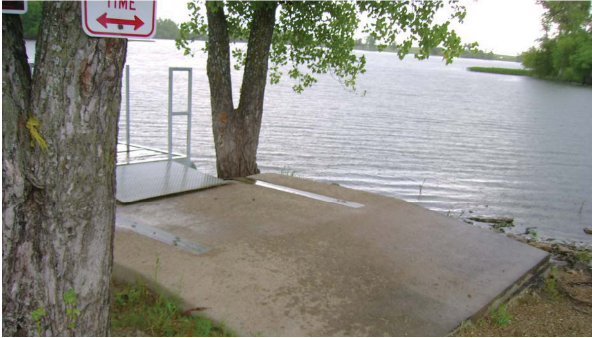
Figure 3a. View of concrete pad benchmark site.
