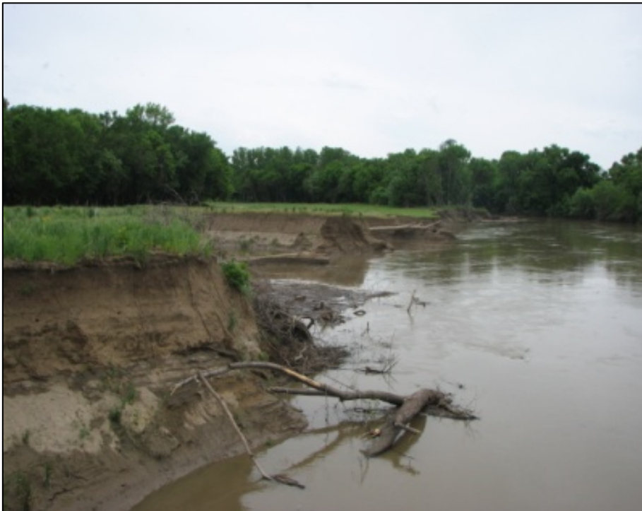
Figure 8. Area above scour pool looking downstream.
