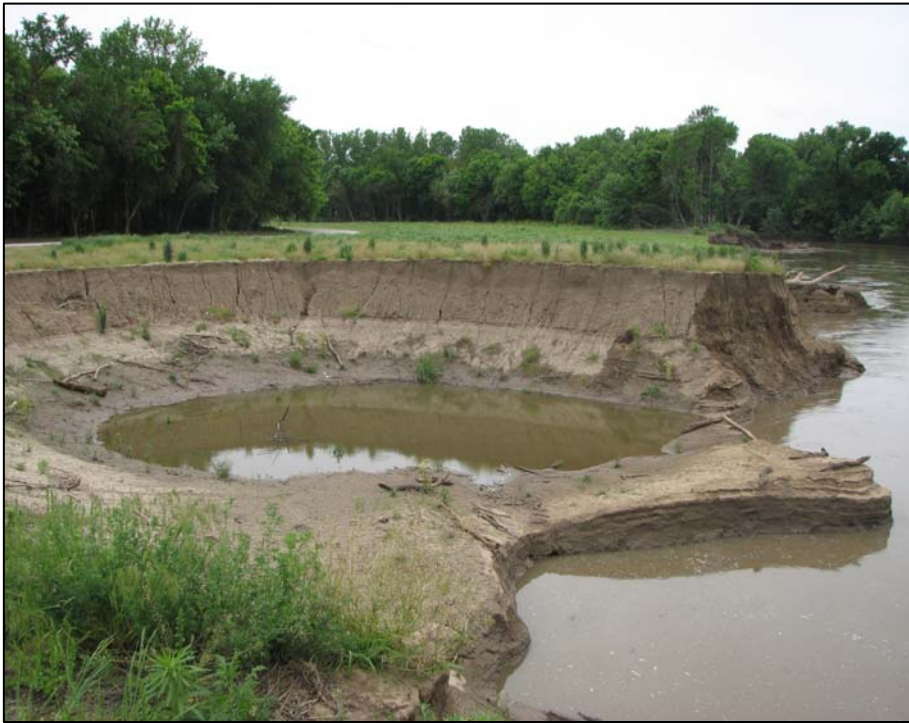
Figure 7. A large scour pool caused by the 2007 flood, it is located at the red dot in Figure 4 (b).
