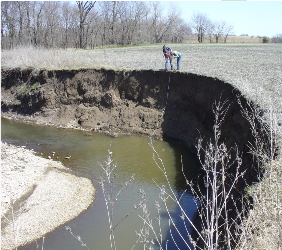
Figure 4. Streambank Height Measurement on the Neosho River
