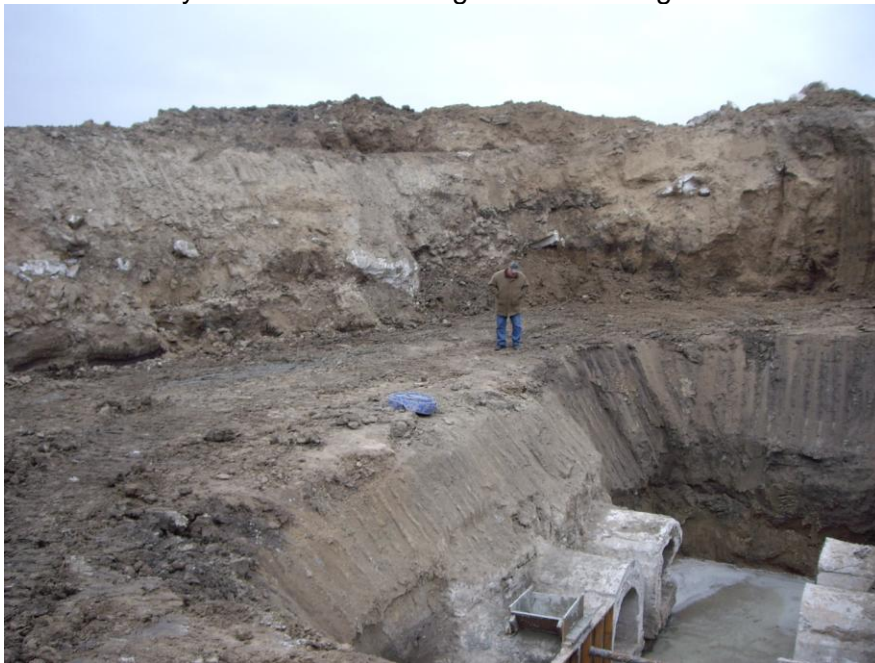
Hole in center of Lake McKinney Dam for control gates work.
