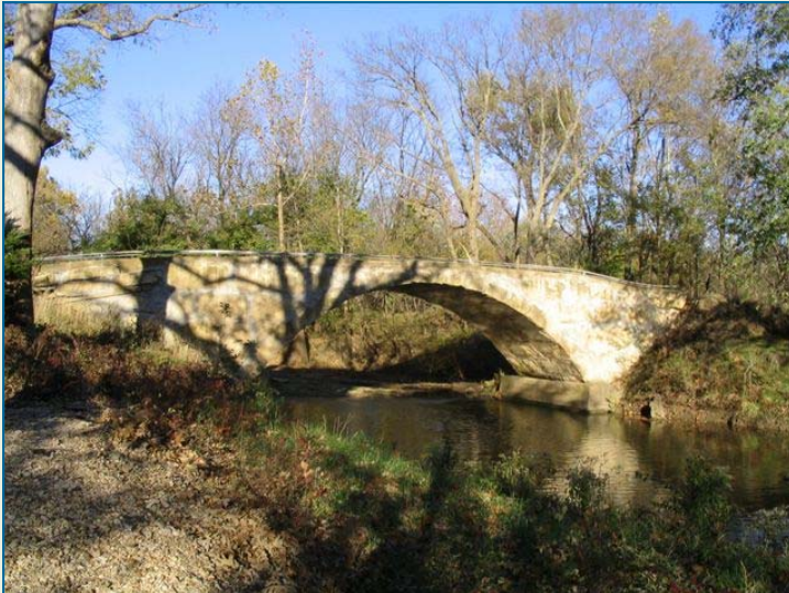
Stone Bridge over Badger Creek, Cowley County Photo courtesy Kansas Geological Survey
