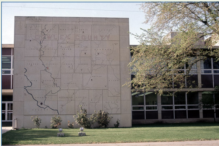
Cowley County Courthouse, Winfield, KS Photo courtesy Kansas Geological Survey.
