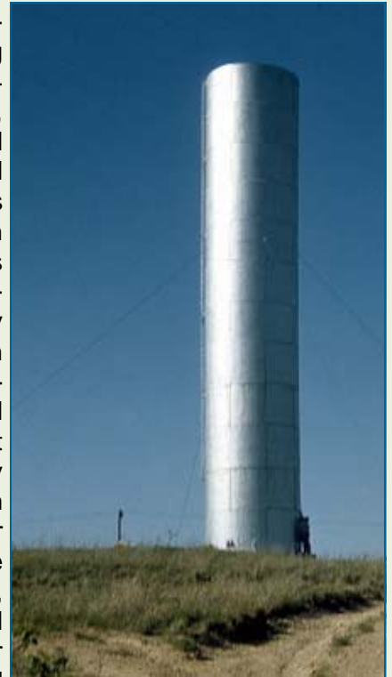
Water Tower South of Cherryvale. Photo courtesy KGS.
