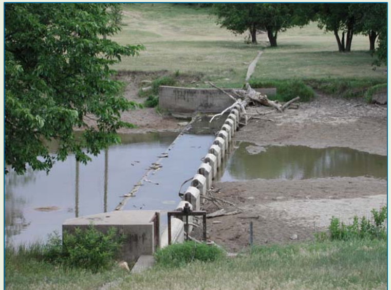
Smoky Hill River Dam at Pfeiffer. Photo by Kansas Water Office
