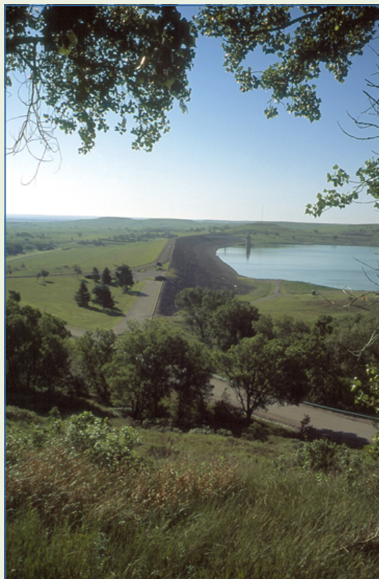
Wilson Reservoir Dam on Saline River. Photo courtesy Kansas Geological Survey.
