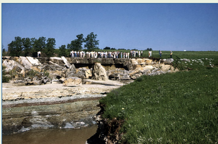
Lake Kahola spillway Photo courtesy Kansas Geological Survey.
