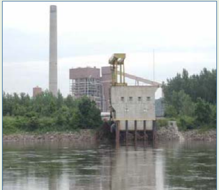
Nearman Creek Power Station
