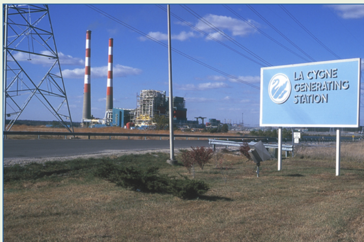
La Cygne Generating Station. Photo courtesy Kansas Geological Survey
