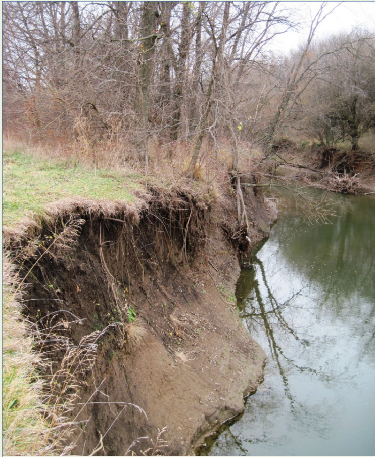
Figure 7. Elm Creek Streambank Erosion Site; Estimated sedimentation rate at 766 tons/yr
