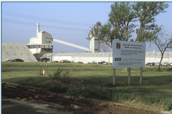
Salt Mine near Lyons, Rice County. Photo courtesy Kansas Geological Survey.
