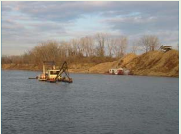
Dredge, Mile 13. Friends of the Kaw Photo
