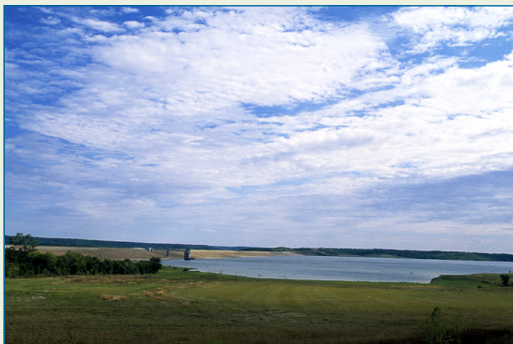
Clinton Dam, on the Wakarusa River. Photo courtesy KGS.
