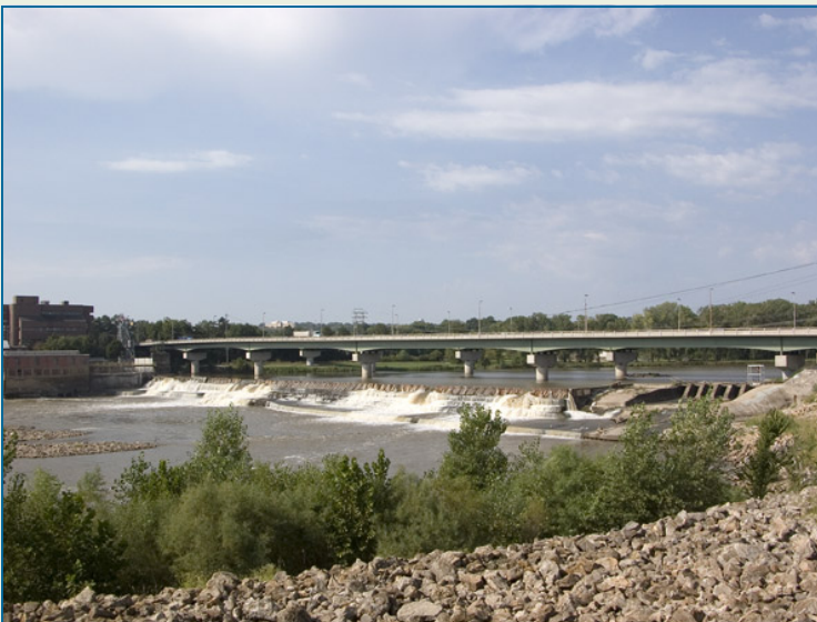
Bowersock Dam on the Kaw River at Lawrence. Photo courtesy Kansas Geological Survey
