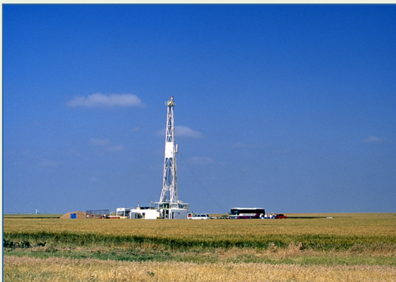
Drilling rig, Anadarko Oil and Gas, Seward County. Photo courtesy Kansas Geological Survey.
