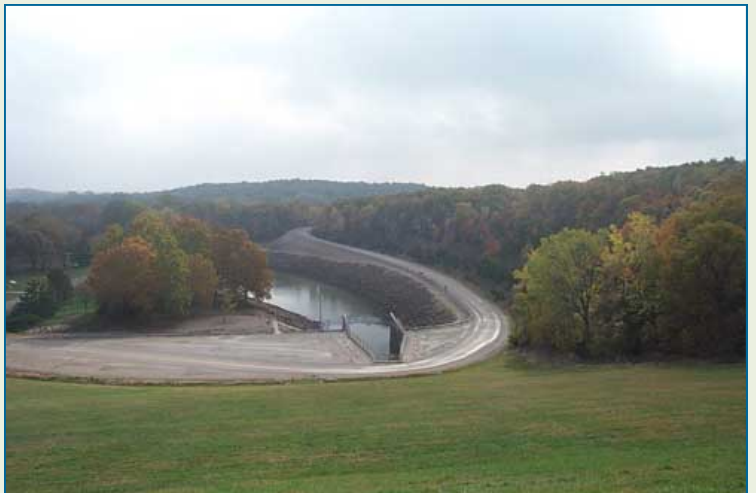
Pomona Reservoir Outlet Channel. Photo by Corps.
